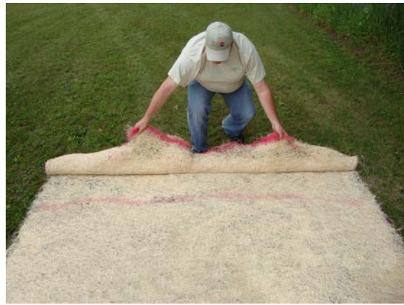
Figure 2. Pull end of RECP along red line.
