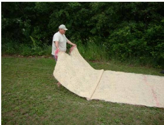
Figure 3. Walk RECP back, while holding near both corners.
