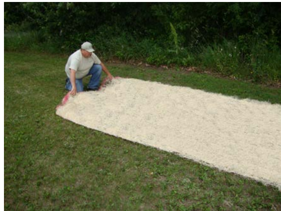
Figure 4. Properly position unrolled RECP for installation.
