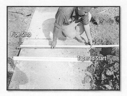
Place a piece of pipe next to the Sidewalk Sleever with one end touching the "pipe stop" and mark, with your finger, where the pipe just meets the tapered end. Then cut the pipe at that point. If the pipe is past the tapered end this will allow dirt to enter the pipe during installation.
