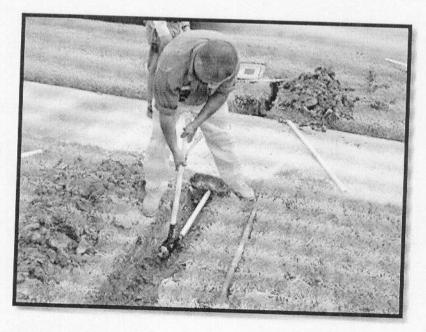
While straddling the trench, use a 16 pound sledge hammer to impact the Sidewalk Sleever under the sidewalk. Continue impacting the tool until the tapered end appears at the other end.
