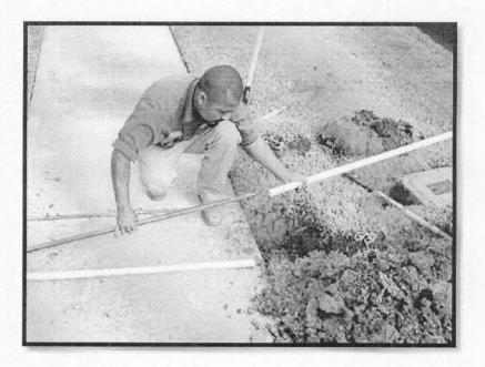
Take the cut pipe (sleeve) and slide it on the Sidewalk Sleever. It is important that the Sidewalk Sleever is clean. Dirt on the tool will make extracting the tool difficult.
