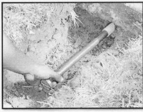
Once the tool and pipe are visible at the other end, simply grab the impacted end of the tool and remove from the installed pipe. If necessary, tap the pointed end of the tool with the hammer to help the Sidewalk Sleever slide out of the pipe.
