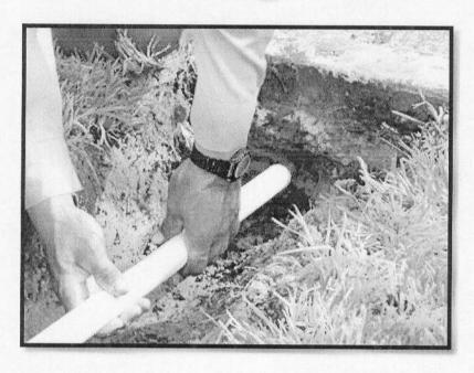
Place the Sidewalk Sleever just under the concrete and tap in a few inches. This will allow the tool to hold itself off the ground making it easier to install and also easier to remove the tool after installation.
