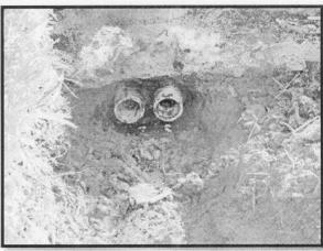
Although soil conditions and experience can determine the speed of the installation, in the example here, the pipe was installed in under 60 seconds. Once the pipe is installed, you can glue on to the pipe or you can use the installed pipe as a sleeve for wires. If more sleeves are needed, just simply repeat the steps and install as many pipes as needed.
