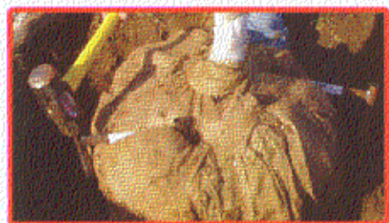
Hit long prong with Sledgehammer
